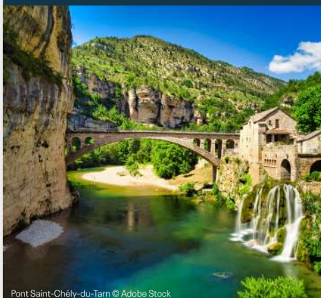
Pont Saint-Chély-du-Tarn © Adobe Stock
